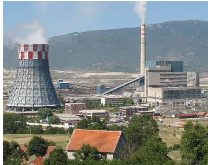
Existing Gacko facility (300 MW)
