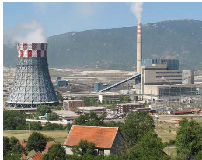
Existing Gacko facility (300 MW)
