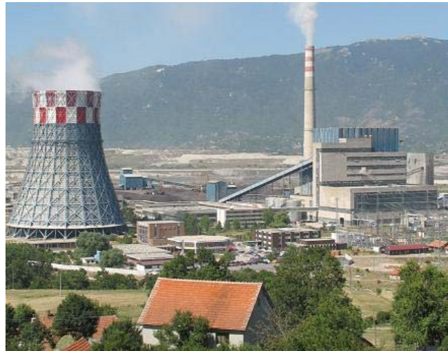
Existing Gacko facility (300 MW)
