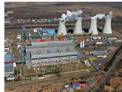
Tušimice power plant after the complex renewal lost its former landmark feature - stack; less exhaust gas is therefore discharged in the air
